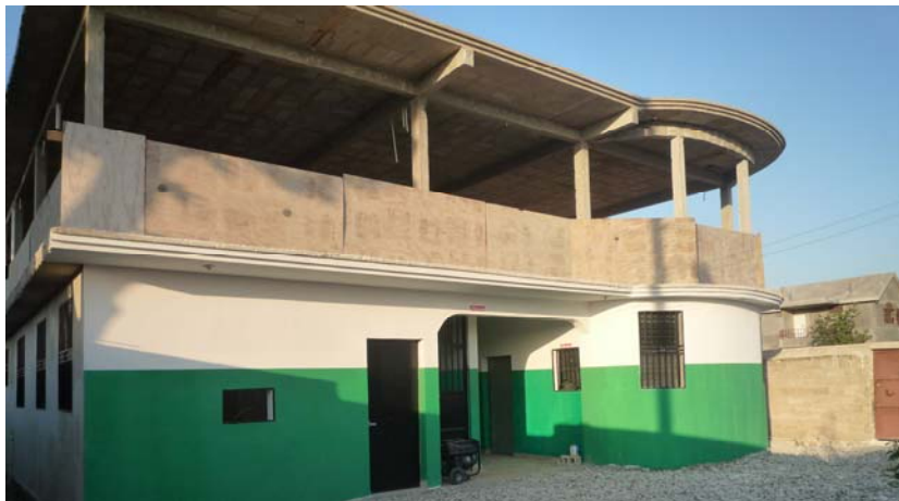
New Satellite/Outpatient Clinic in Leogane (2nd floor in progress)
